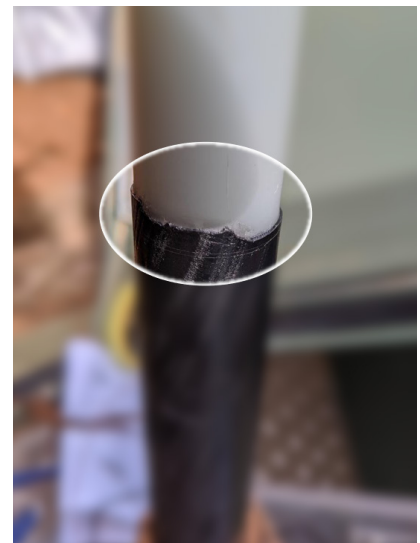
Semi Conductive Layer Cut
