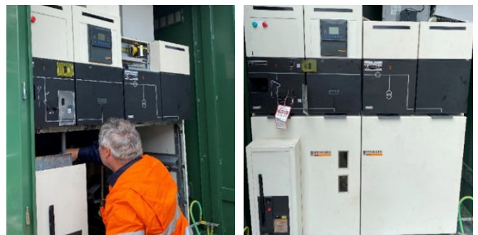
New cabinet installation
